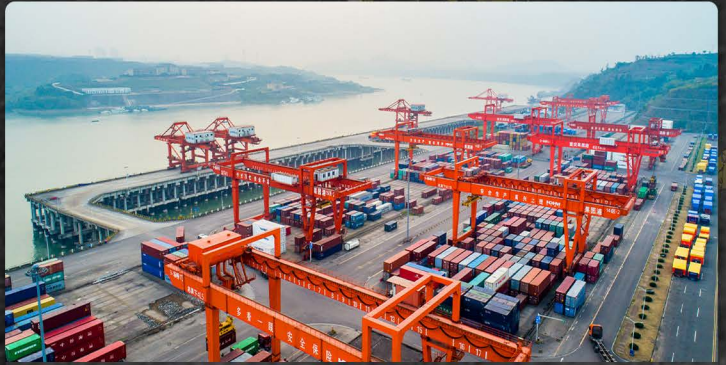
Customs - Cargo Nuclear Radiation Inspection
